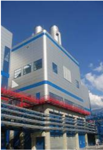
Process exhausts 580 000 m 3 /h
